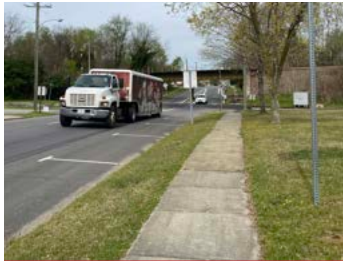
Sidewalks on W 3rd St in Downtown Weldon
