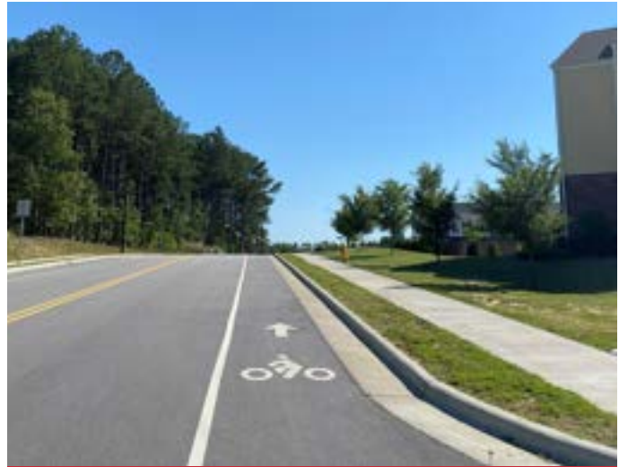
Bicycle lane on Granite Falls Blvd in Rolesville, NC
