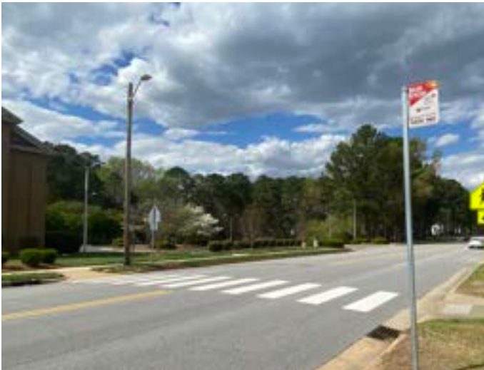
High-visibility mid-block crosswalk on Aversboro Rd in Garner, NC
