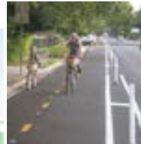
Example of protected bicycle lane with flex posts
