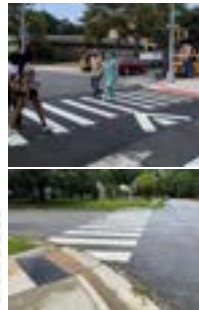
Example of high-visibility crosswalk markings
