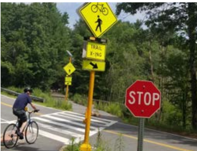
Rectangular rapid flash beacon along a trail
