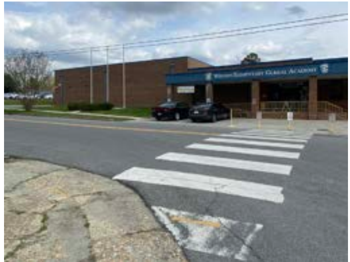
High-visibility mid-block crosswalk on Washington Ave in Weldon
